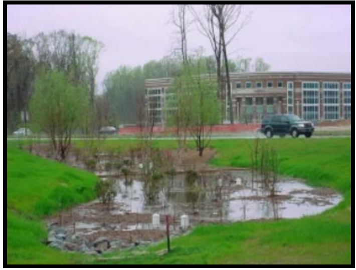
Typical Bioretention Area
